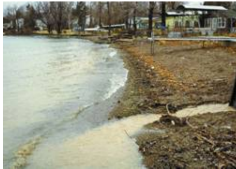
Streambank & Shoreline Erosion
