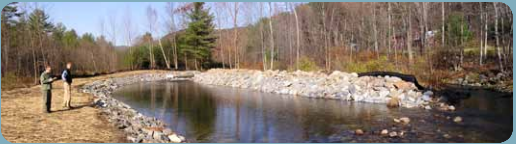
LGA Lake Saving Project: Sediment retention basin on Hague Brook.
