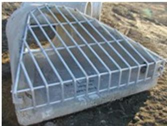
Pictured: Debris guard for a culvert
